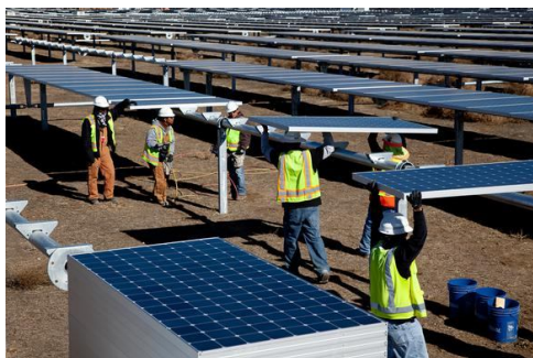
Workers build SunPower's California Valley Solar Ranch. Image source: SunPower.
